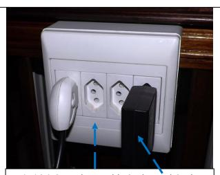
4x164-2 sockets with 3 pin and 2 pin plugs accommodated in the new socket. Up to 6 are possible in one box. Note no switches.
