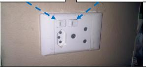
This shows a combined flush mounted double socket consisting of 1x164-2 and 1x164-1 which is a permitted option as are the switches.
