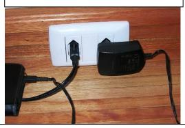
THESE FIXED MULTI SOCKETS DO AWAY WITH DANGEROUS MULTI ADAPTORS. UN-SWITCHED SOCKETS ARE GENERALLY SAFER THAN SWITCHED SOCKETS.
